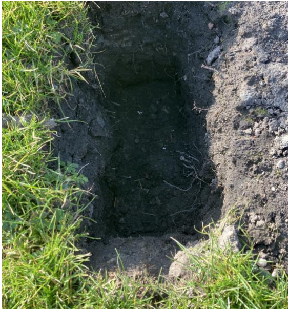
Dig a hole +/- 30 cm wide, to the desired measuring depth
