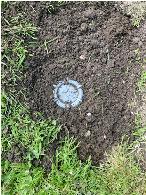
Step 4 & 5. Replace the soil and compress to original soil compaction till the surface is even. DO NOT cover Poseidon City with more than 2,5cm of dirt/stone/wood/etc...
