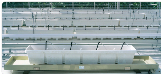
Figure 3. Level installation on the supporting base, drain sensor on the run-off side.
